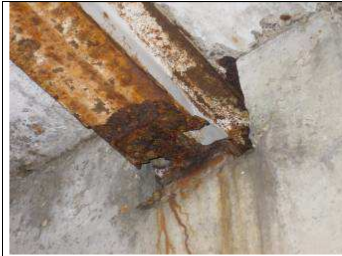
Photo 1: Beam end damage found during December 2014 inspection of Parking Garage C.
