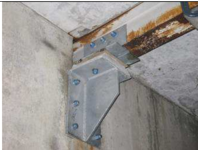
Photo 3: Beam end repair in Parking Garage C completed by Christy-Foltz in April 2015. The deteriorated section was cut out and new structural steel was bolted in place with a structural steel support installed to hold the beam in place.
