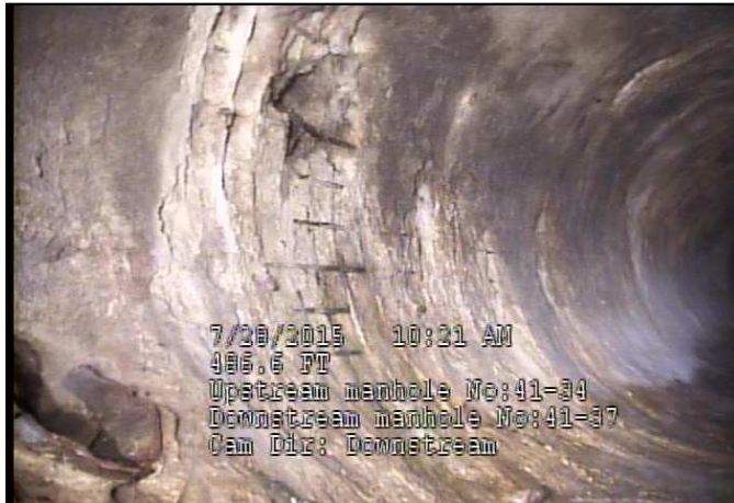
1. Pipe wall deterioration with reinforcement exposed. East of Oakland south of Eldorado.
