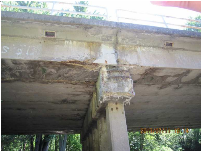
Photo 6: Spalling with exposed reinforcement at the south end of the West Pier cap.
