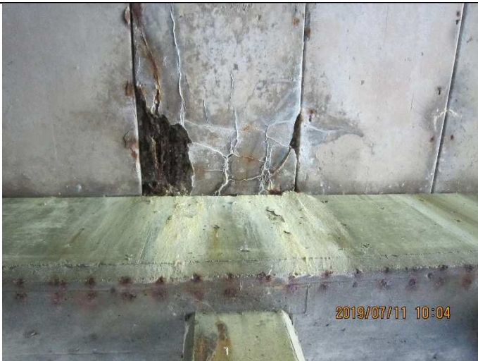
Photo 5: Map cracking at the east end of Beam 6 in the West Span has developed into a spall, exposing 3 strands with one of them severed.
