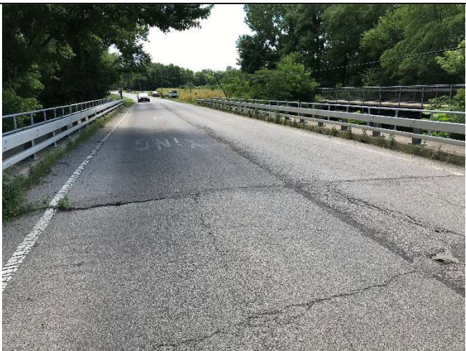
Photo 9: Pavement condition at the west end of the bridge. Centerline is raveling. Some settling past the bridge end.
