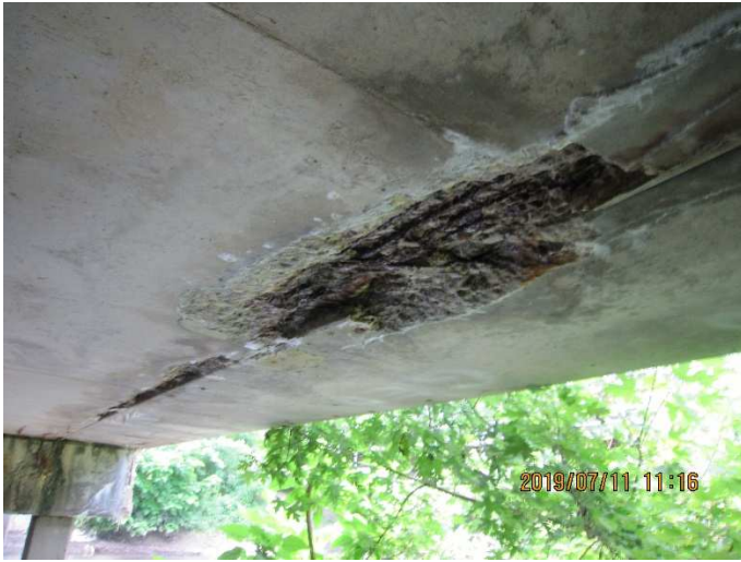
Photo 4: Corners of beams 10 and 11 near midspan of West Span, spalled with 5 exposed strands. 3 of them broken.
