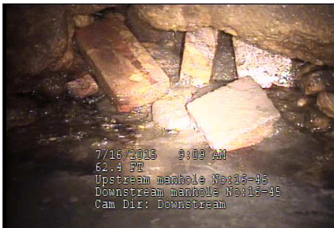
5. Failed section with bricks and backfill visible. Near Pine / Marietta.
