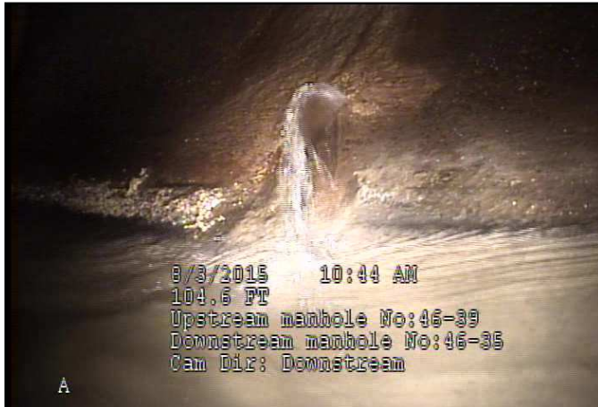
3. Infiltration at a deteriorated joint. Fairview Park.
