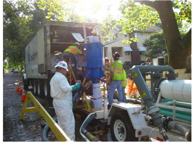
Inserting the liner into the pipe.
