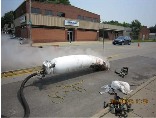
Heat curing of felt tube liner.
