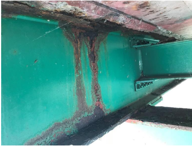
Pack rust on south beam near cross beam. Some rusting on cross beam
