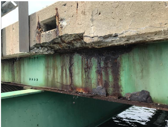
Spalling and cracking around scupper. Heavy pack rust on upper beam flange.
